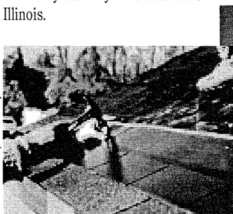
Detail of the installation of a United Solar Systems Corp. amorphous silicon PV roofing shingle.
